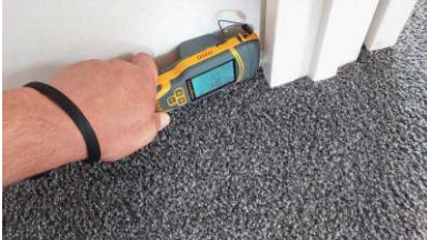
Base level moisture test internal wall.
